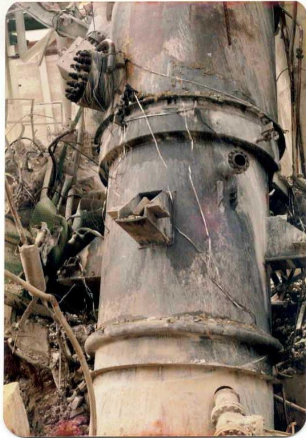
Stripper found after accident
